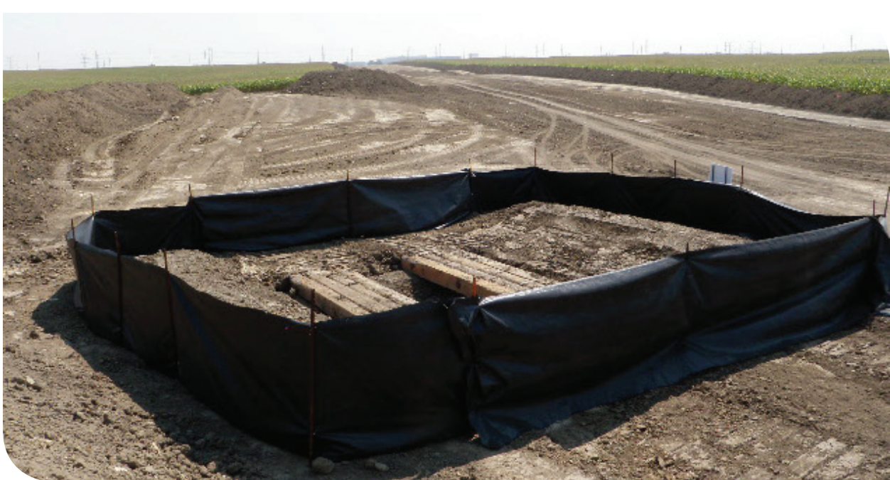
Cleaning station at construction site.
