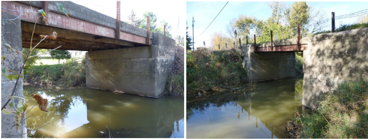
Figure 1 – North (left) and south (right) portals of bridge structure C001. (LSHC 2013) 040, 049
