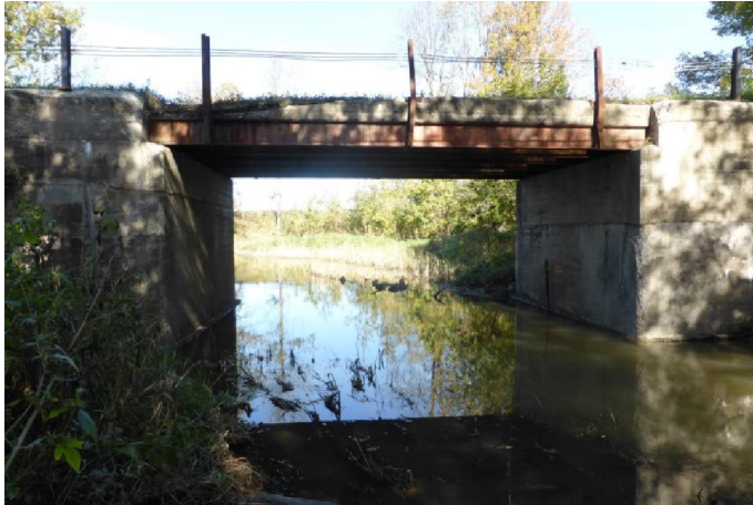
Figure 9 – South portal of Bridge C001. (LSHC 2013) 876
