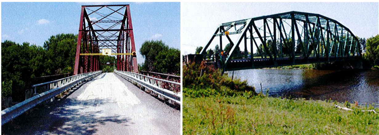
Figure 11 – SP020 “Chartrand Bridge” (1930, left) and C005 “Touchette Bridge” (1950, right) are through-truss bridges over the South Nation River in The Nation Municipality. (Keystone, 2013)
