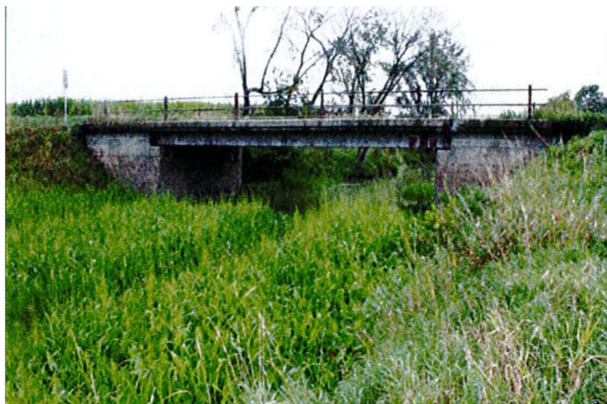
Figure 13 – SP003, built 1960 over the West Scotch River, is a concrete slab on steel girder, similar to C001.
