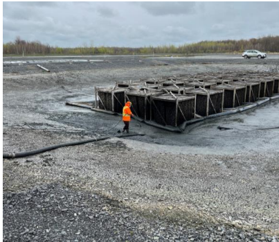
Biocord™ Desludging
