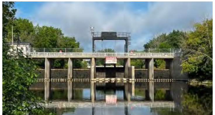
Chesterville Dam, Township of North Dundas
