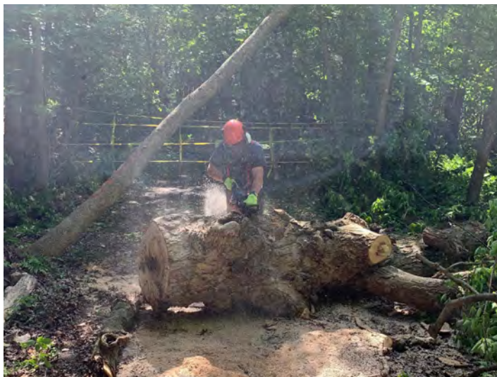
Cleaning up conservation areas following the derecho storm
