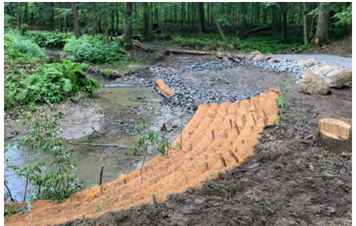
Shoreline restoration, Township of Russell
