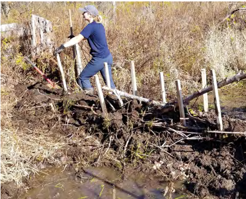
Building beaver dam analogs for wetland restoration, Township of Alfred and Plantagenet
