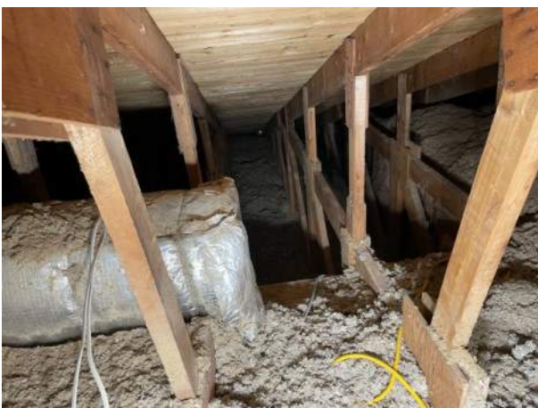
Photo #5: Trusses At Built-Up Beam Location
