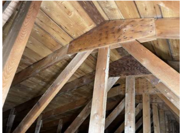
Photo #8: Truss Members At Center Node Point
