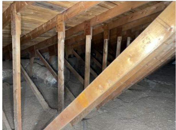
Photo #10: Truss Members
