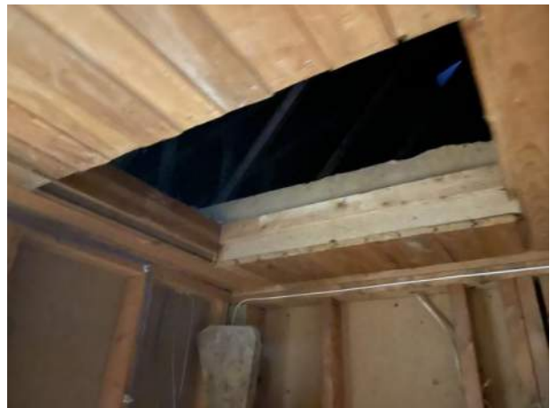
Photo #4: Planking On Underside of Trusses
