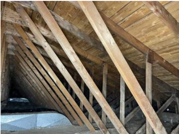
Photo #9: Truss Diagonal Webs
