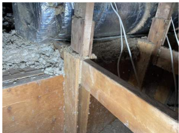
Photo #6: Trusses At Built-Up Beam Location
