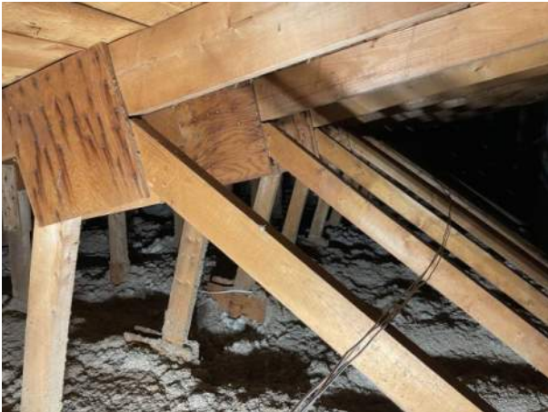
Photo #7: Truss Members At Node Point
