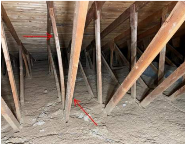
Figure 2: Swaying/Bending of Truss Members
