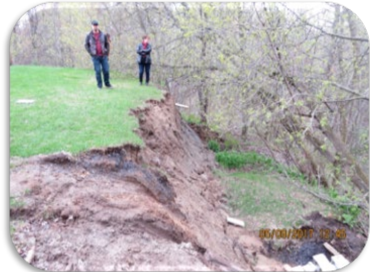
Small-Scale Landslide following unpermitted garage construction, 2017.
