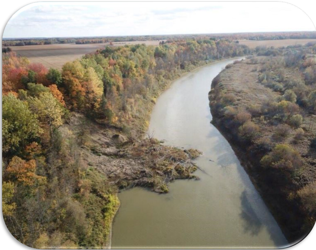
Slump downstream of Wolf Creek, La Nation, Fall 2018.
